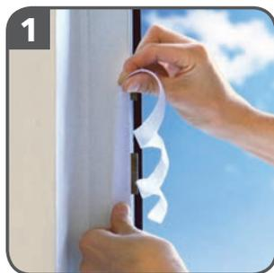
First open the window and clean the surfaces to be bonded from dust and fat on the window frame and casement. Open the Velcro fastener and stick the Velcro strap to the window frame (**side A**).
